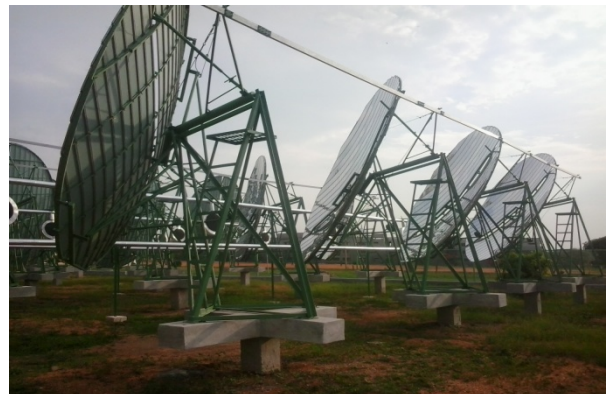
View of Tracking System of Solar Array
