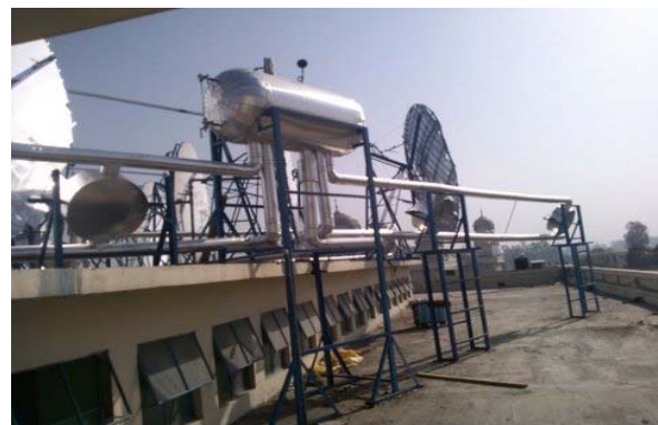
CST system at Gurudwara, Karmasar
