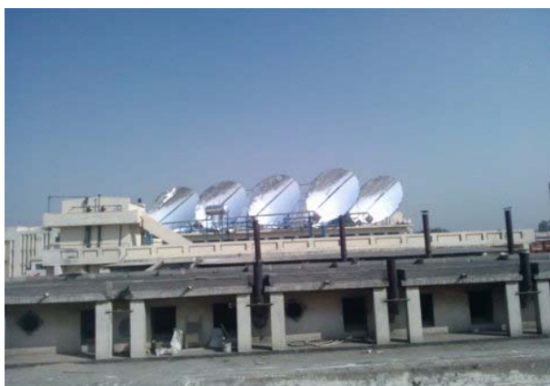
CST system at Gurudwara, Karmasar
