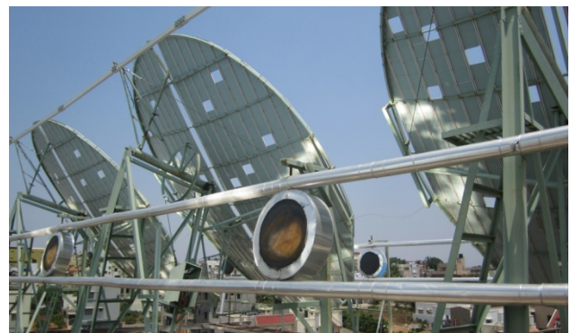
Heat Receiver and running water piping
